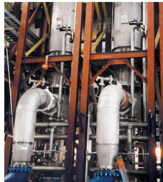
Vertically installed, multi-pass membrane modules in a multi-stage system design. Vertical configuration conserves floor space.
